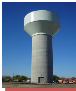
Water System Development
